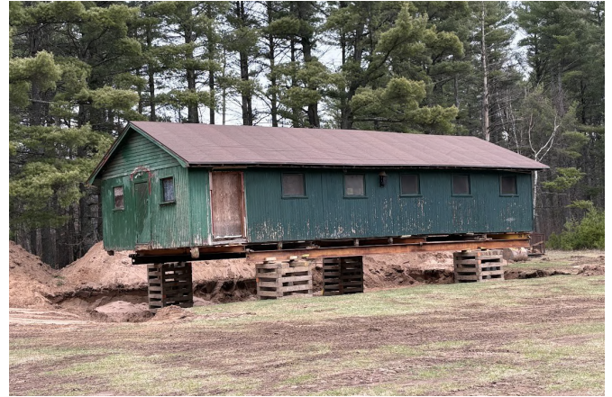
A foundation was dug out and laid before the building could be set in place.
